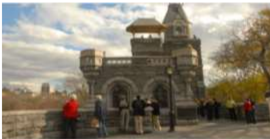
Belvedere Castle, Restored 1983
